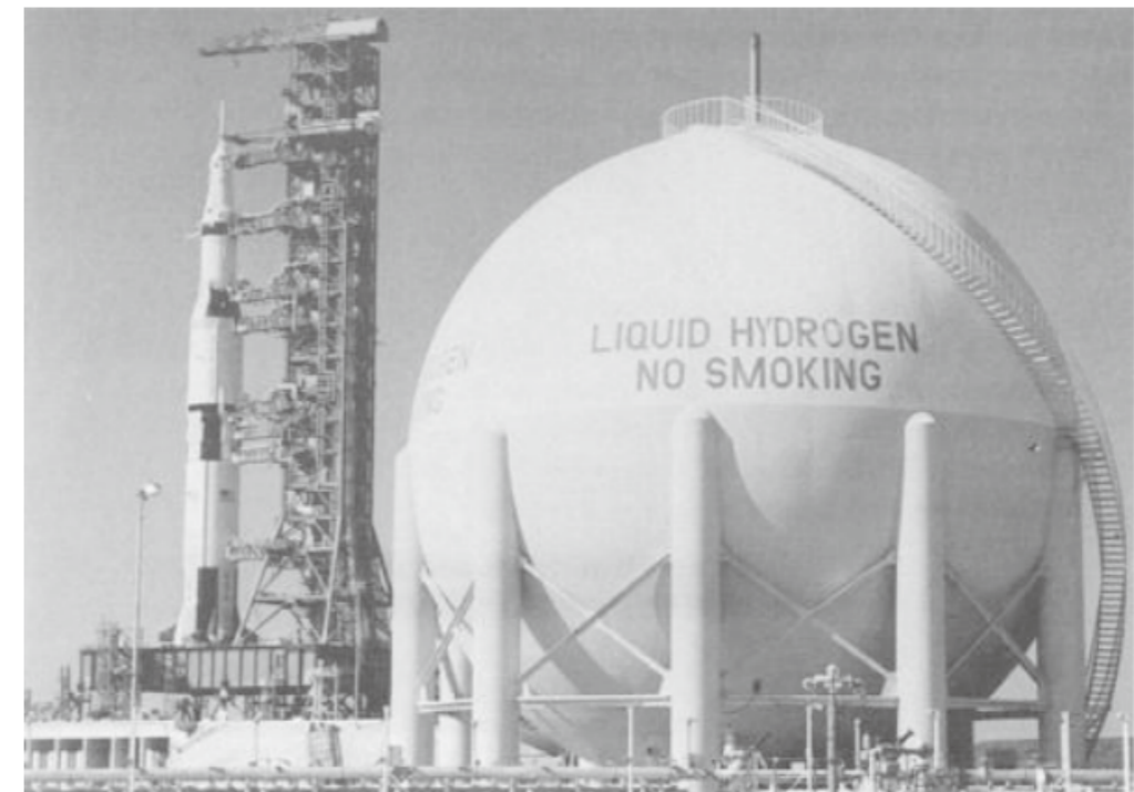
图2 美国航天发射场及其液氢储罐（图源：Laurence Bernard et al. State of the art of LH2 installations and facilities.
